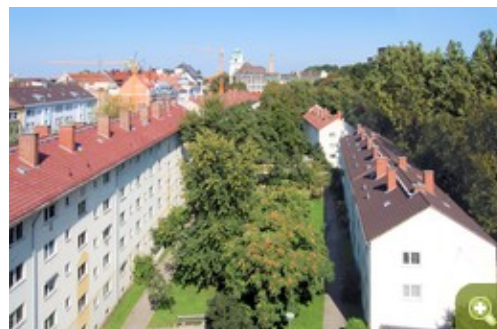
Aerial view of the four blocks of flats © Fraunhofer IBP
